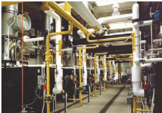
Pictured above is California State University, Long Beach's central plant. 63,000,000 BTU's of low emmissions, high efficiency heating.
